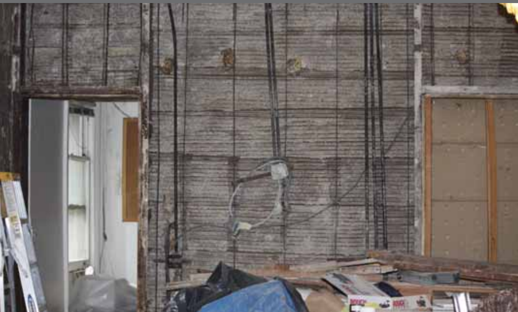
WEST WALL, READING ROOM - BEFORE
